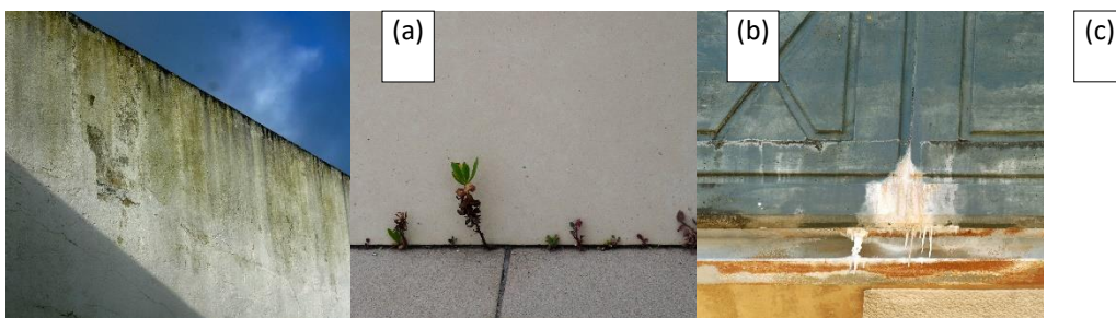
Figure 2. Examples of three types of defects [1]: a) “A-B1 Biodeterioration/biological growth”; b) “A-B2 Vegetation growth”; c) “A-B3 Efflorescence/cryptoflorescence and carbonation”
